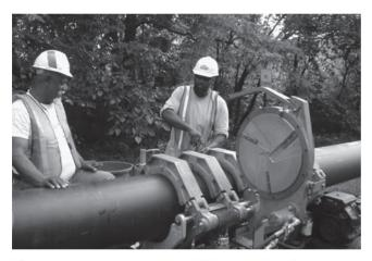
Figure I Joining Large Diameter PE Pipe with Butt Fusion
