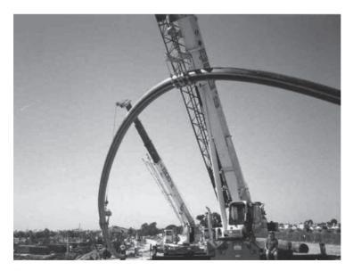
Figure 3 Butt Fused PE Pipe "Arched" for Insertion into Directional Drilling Installation
