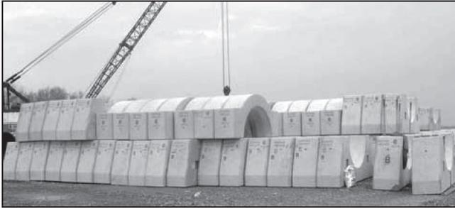
**Figure 3** Two-piece Concrete Anchors in Storage at Marine Job-Site
