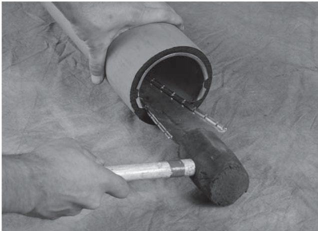
Figure 12 Install Split Ring Stiffener in PE Pipe
